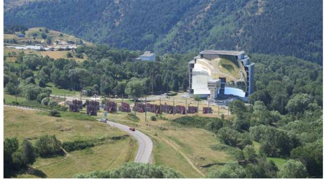
Fig. 1. PROMES laboratory at Odeillo, southern France, showing the 1MW parabolic mirror (north part of the building) and the heliostat field. Smaller size solar furnaces are located in the building at its southern part.
